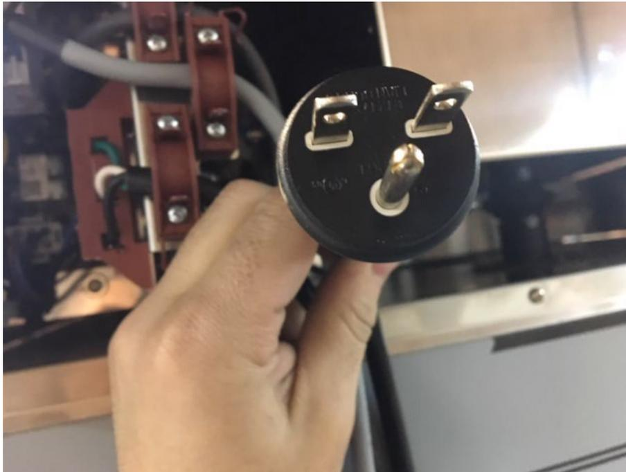
Each Bakerlux oven needs a dedicated circuit. The amperage will vary depending on the power of the model, and if ovens are installed on single phase or three phases.
