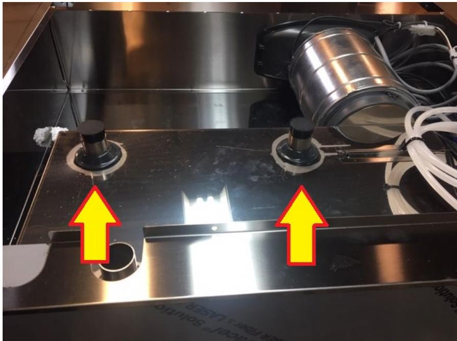
Install the small rubber pipe to join the top oven exhaust with the hood.
